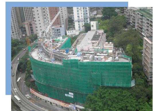
Latest elevation view of the constructed Main Building
