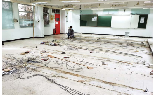
▲ Site clearance at a classroom of Caritas Sha Tin Social Centre
